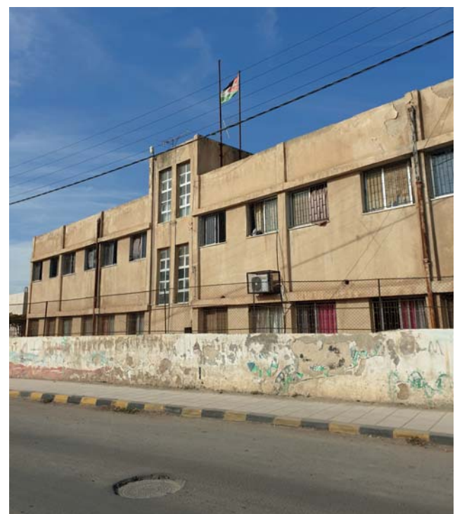
An Image Showing that there is a Sewerage Network in the Neighbourhood (UN-Habitat, 2021)
