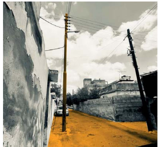
Deteriorated Street, Electrical Poles
