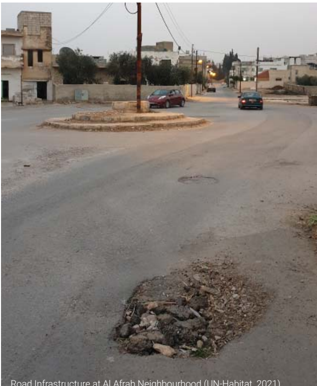
Road Infrastructure at Al Afrah Neighbourhood (UN-Habitat, 2021)
