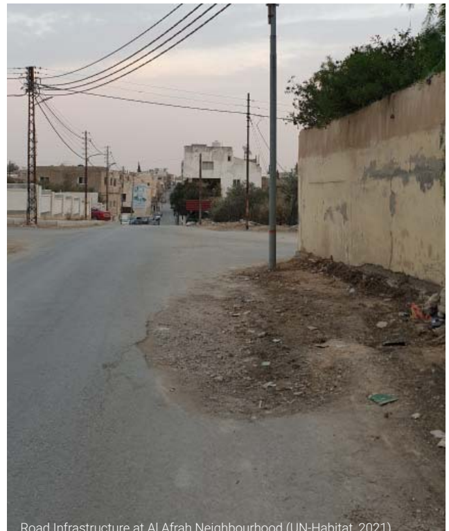
Road Infrastructure at Al Afrah Neighbourhood (UN-Habitat, 2021)
