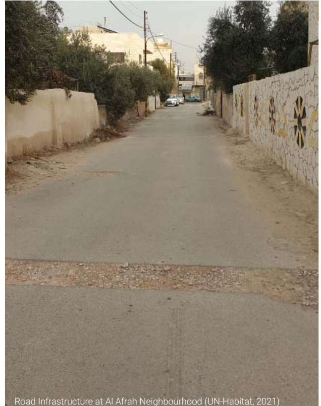
Road Infrastructure at Al Afrah Neighbourhood (UN-Habitat, 2021)
