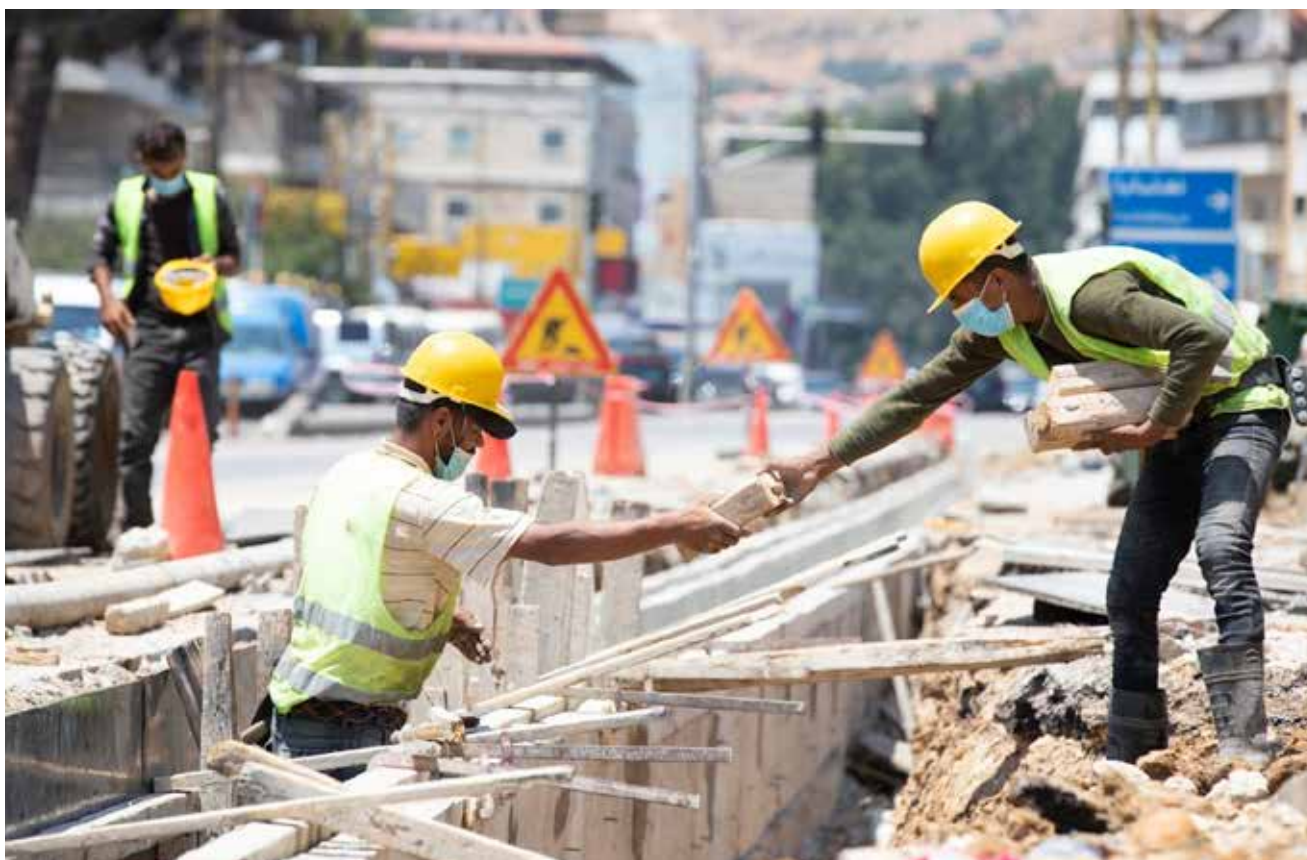
Construction of stormwater canals in Chtoura prevent cross-contamination and flooding during heavy rains.
